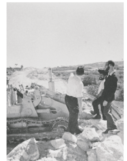
Rav Levinger next to the tractor that will pave the way to the beginning of the construction of Kiryat Arba. 1970. Photo: Gershon Ellinson. All rights reserved
